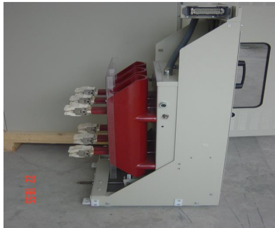
Medium voltage circuit breaker
