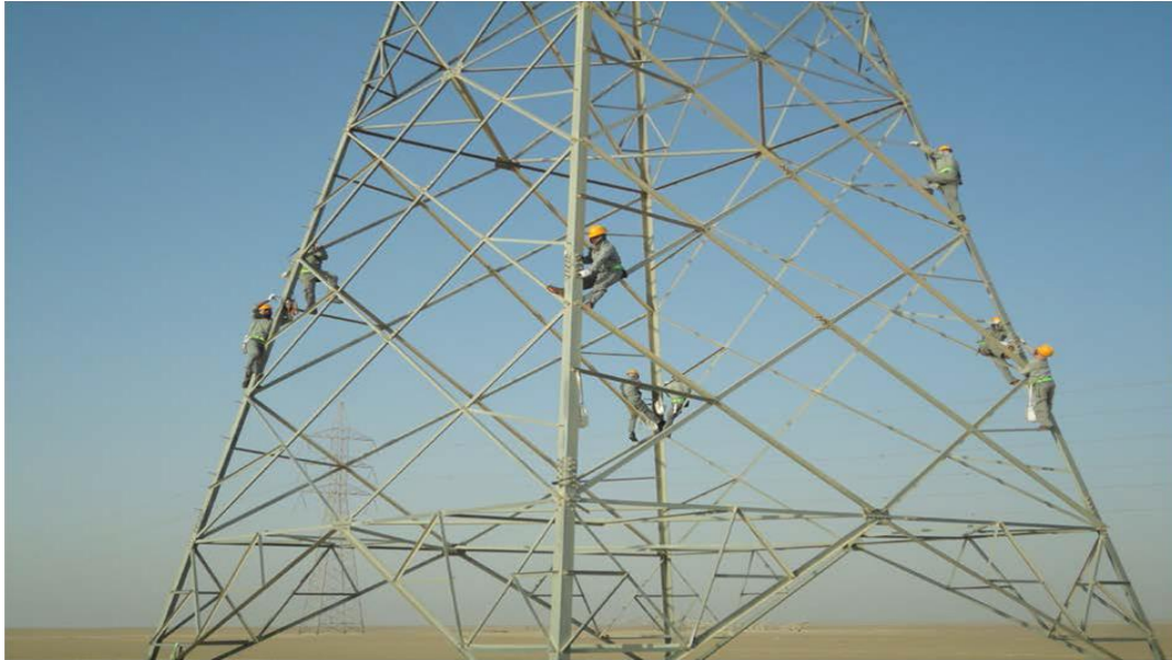
Tower erection
