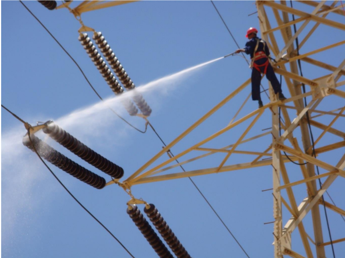
Under voltage cleaning
