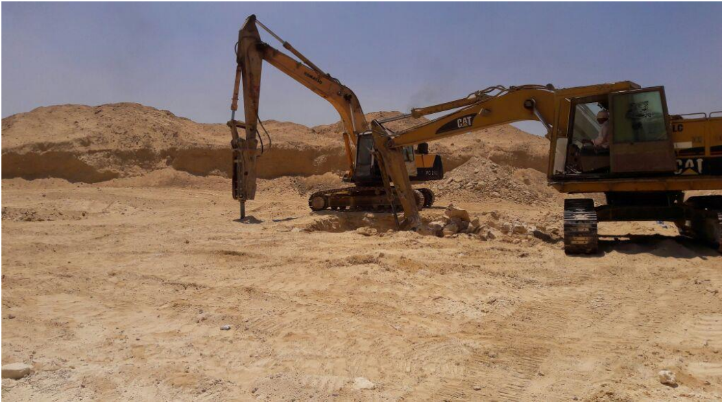
Excavation in stone soil
