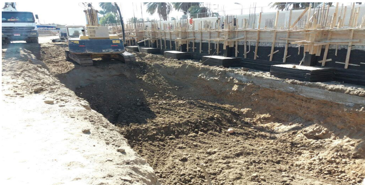
TEMA Civil works AIS 66/11 KV Substation
