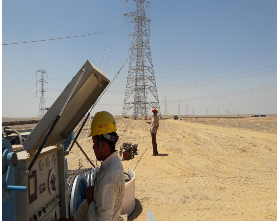
Stringing of conductors
