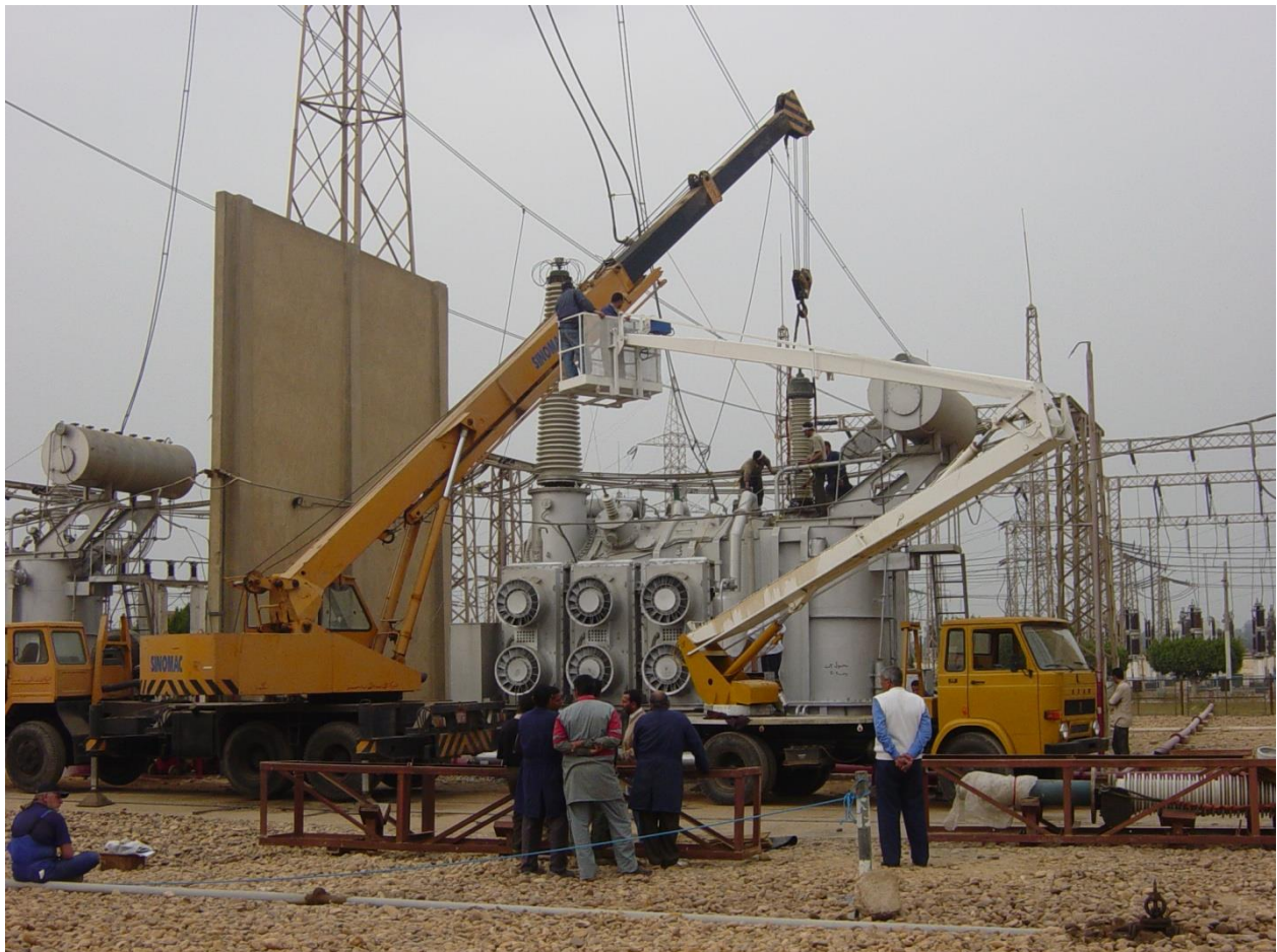
Repair of 500 KV autotransformer at Cairo 500 S/S
