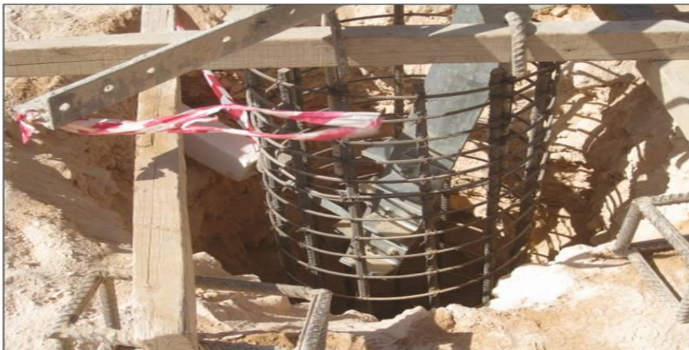
Pile with steel
